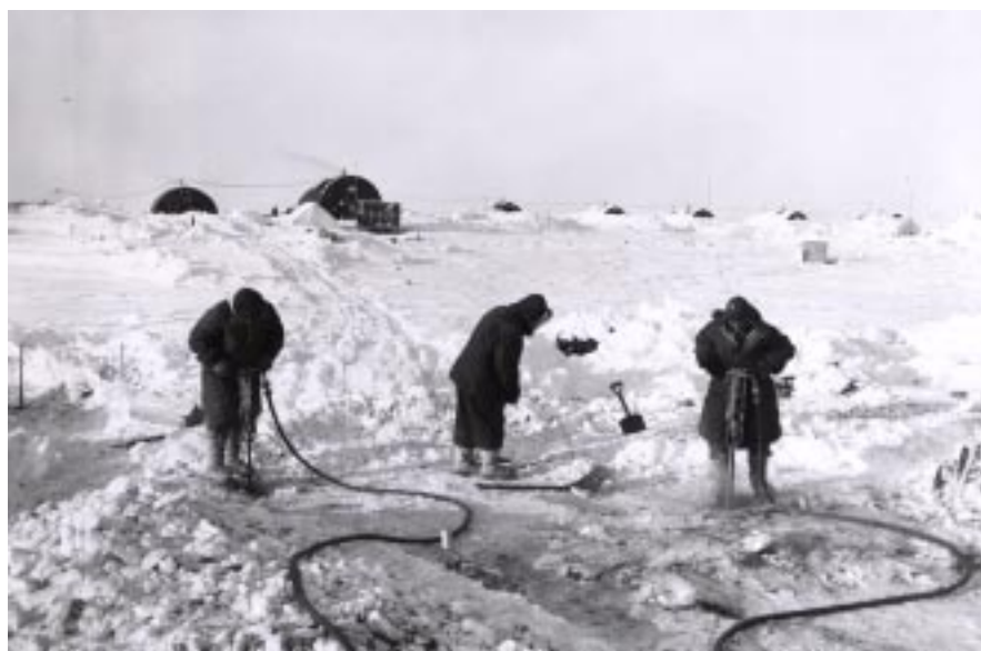
Paging Nanook. Construction workers drill foundation piers for a DEW Line building on Canada’s Baffin Island, north of the Arctic Circle. Temperatures at such sites could hit 65 degrees below zero.
