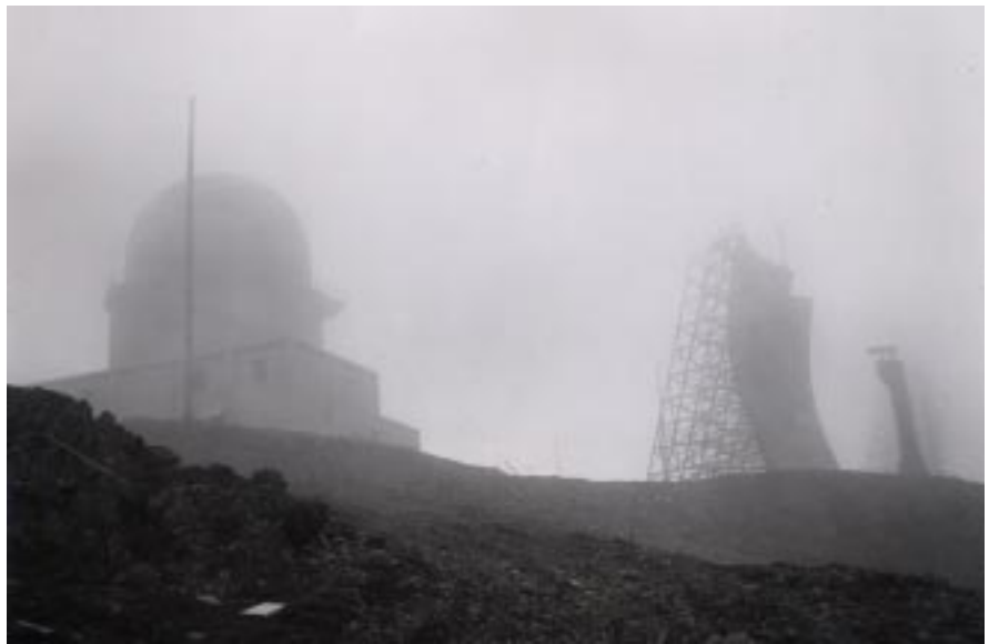
Fog of Cold War. In the Aleutians, heavy fog envelops a DEW Line station (left) and two antennae of a later communications system, dubbed White Alice. The Soviet bomber threat faded, and so did the DEW Line.
