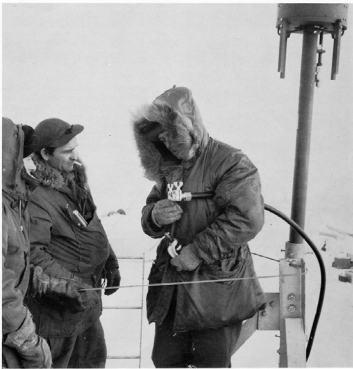
Rigger Mechanics at Work Atop 30' Dish
