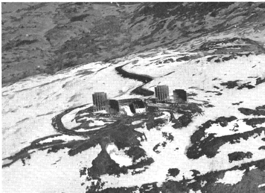
White Alice Station at Pillar Mountain. Shows 60-foot antennas and building. Note access road in center background.
