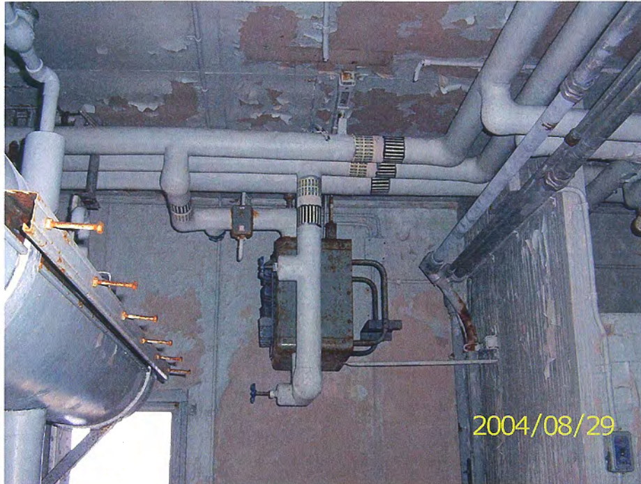
Photo 49 Typical piping insulation and paint condition – Module Train
