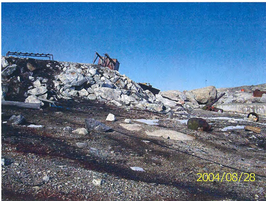
Photo 34 Staining below Garage, looking north east
