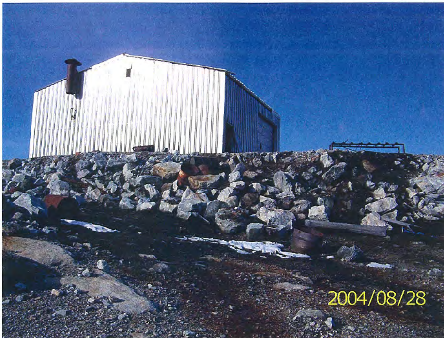
Photo 33 Staining below Garage, looking north
