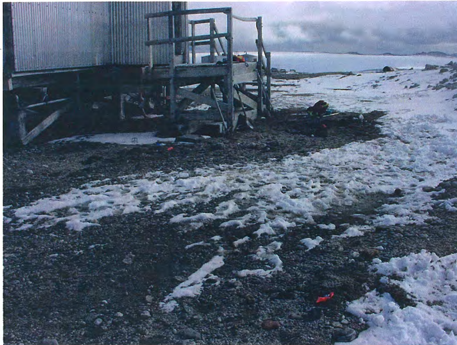
Photo 23 Metal impacted at west end of Modular Train
