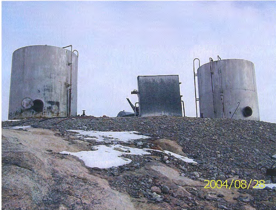
Photo 39 POL Storage Facility, looking north
