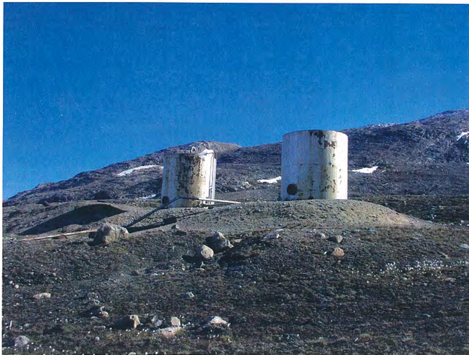
Photo 2 Beach Area POL tanks, looking southeast
