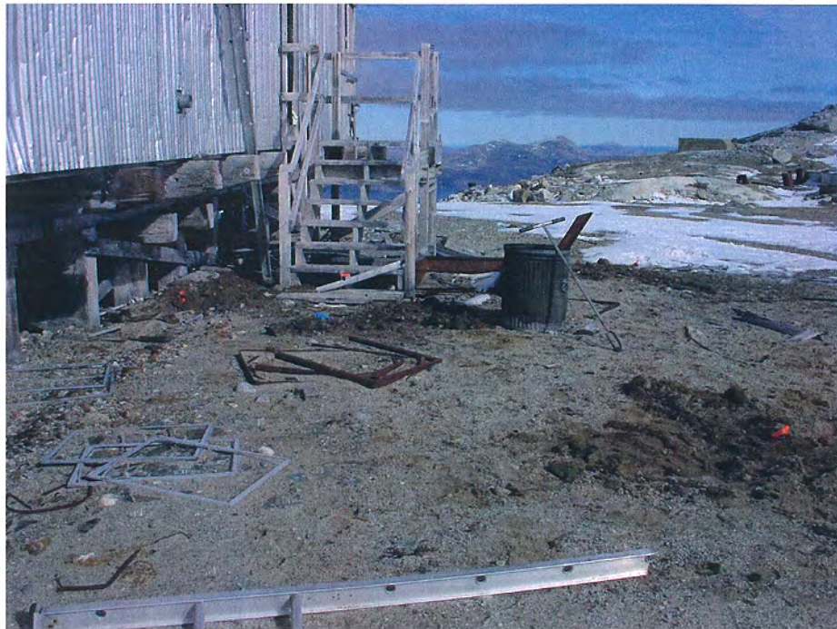
Photo 22 PCB impacted area on south side of Module Train
