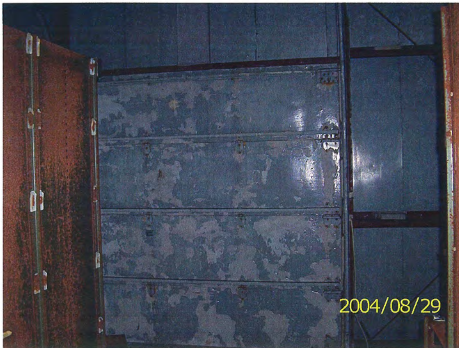
Photo 52 Overhead door and exterior wall cladding – Warehouse
