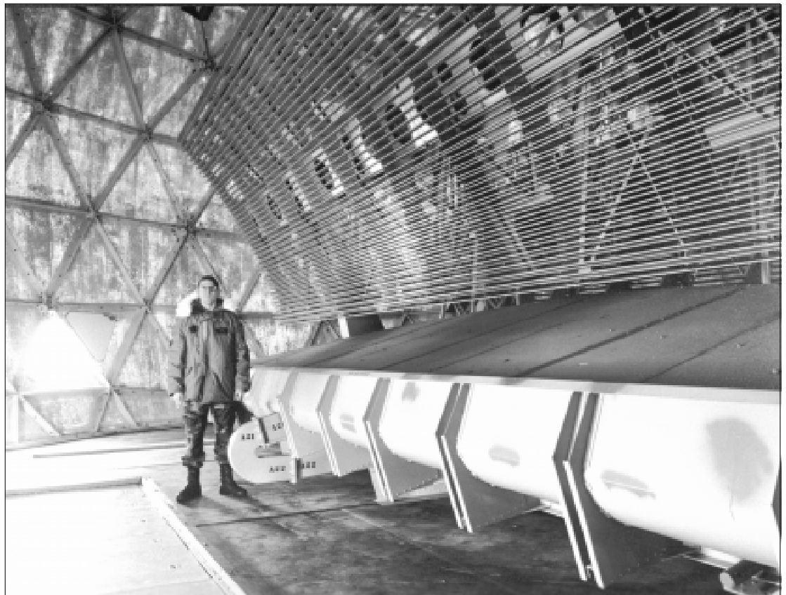
USAF Captain Joseph A. Miller beside the radar array in the geodesic dome, BAR-1, April, 1993. Johnson collection, Parks Canada.
