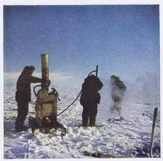
It took live "steam-pointing" to drill holes in ice and "permafrost" to set stakes and poles which when set immediately froze fast.
