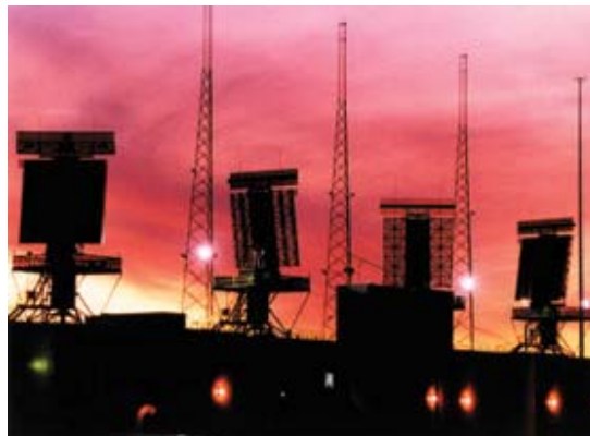
Four FPS-177 long-range surveillance-radar arrays undergo testing at Lockheed Martin's Syracuse, New York, facilities, 2003.
