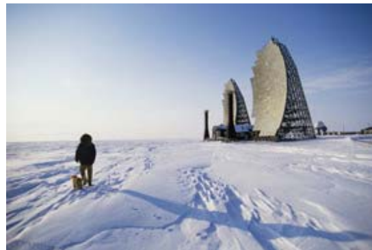
A radar station near the northeast corner of Alaska, once part of the front line of the Cold War.
